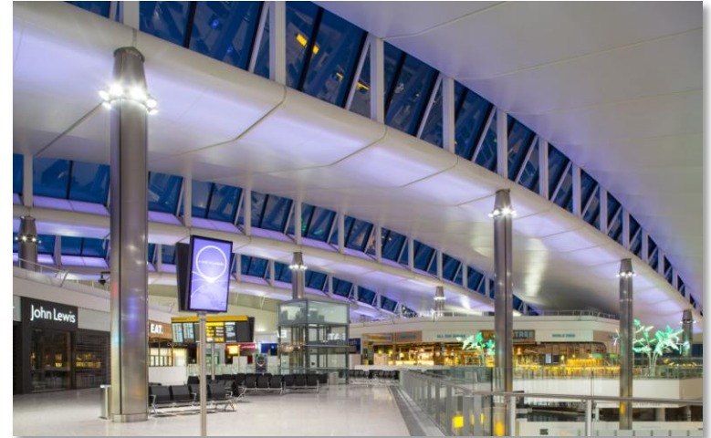
Terminal 2 departure lounge and retail area
