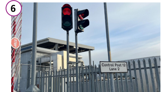
Holding point traffic lights
