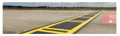
At Heathrow this will indicate a CAT II/III holding point (where there is a separate CAT I holding point ahead).
