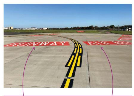
Red paint containing white text stating Runway Designators and 'RUNWAY AHEAD' painted on the taxiway surface prior to the runway holding position. This provides a supplementary visual cue alerting pilots and drivers of an upcoming runway holding position.
