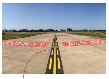
Enhanced markings consist of an additional 15 dashed lines on both sides of the solid taxiway centreline. They are intended to provide an additional visual cue for pilots and drivers approaching a runway.
