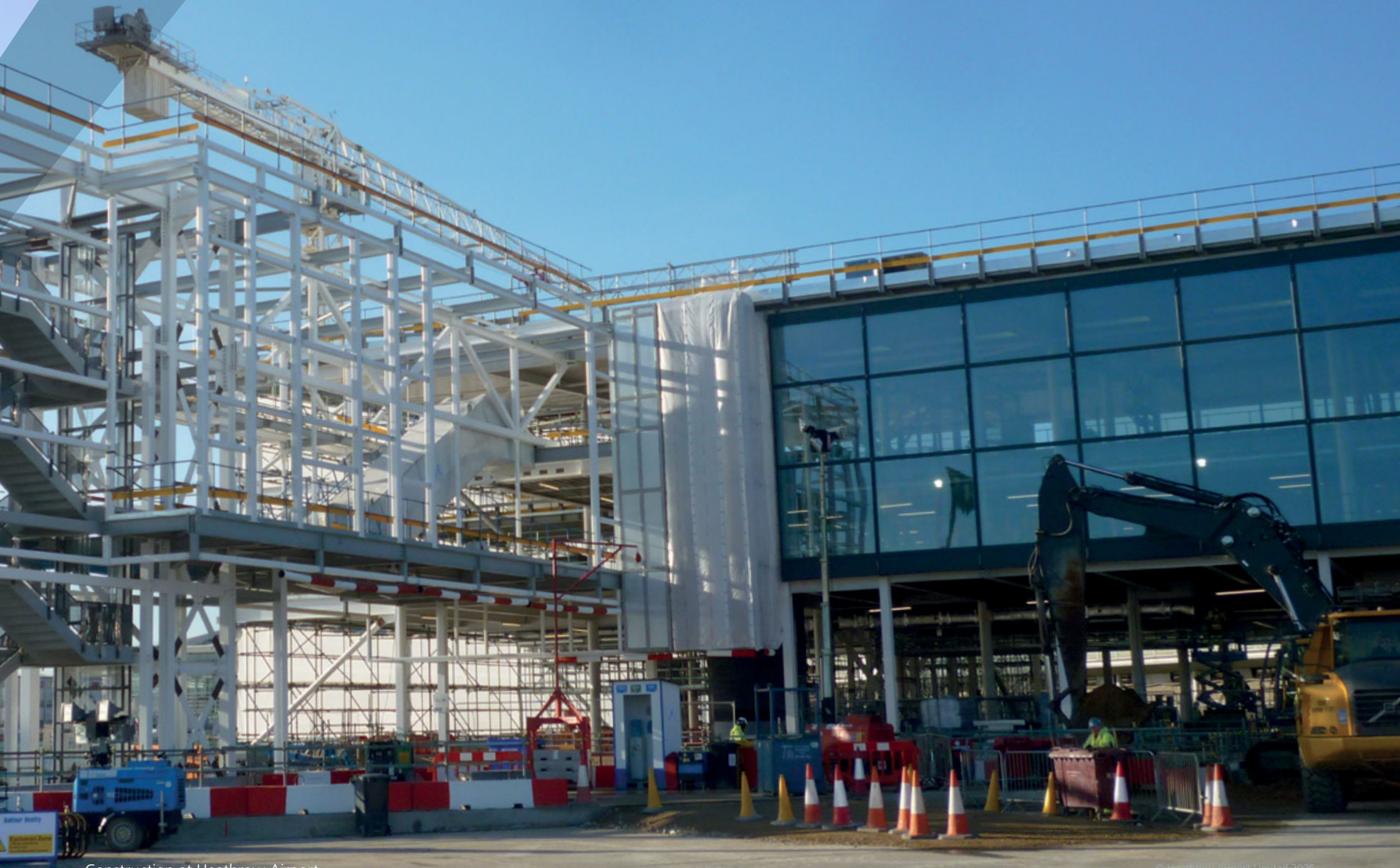
Construction at Heathrow Airport
