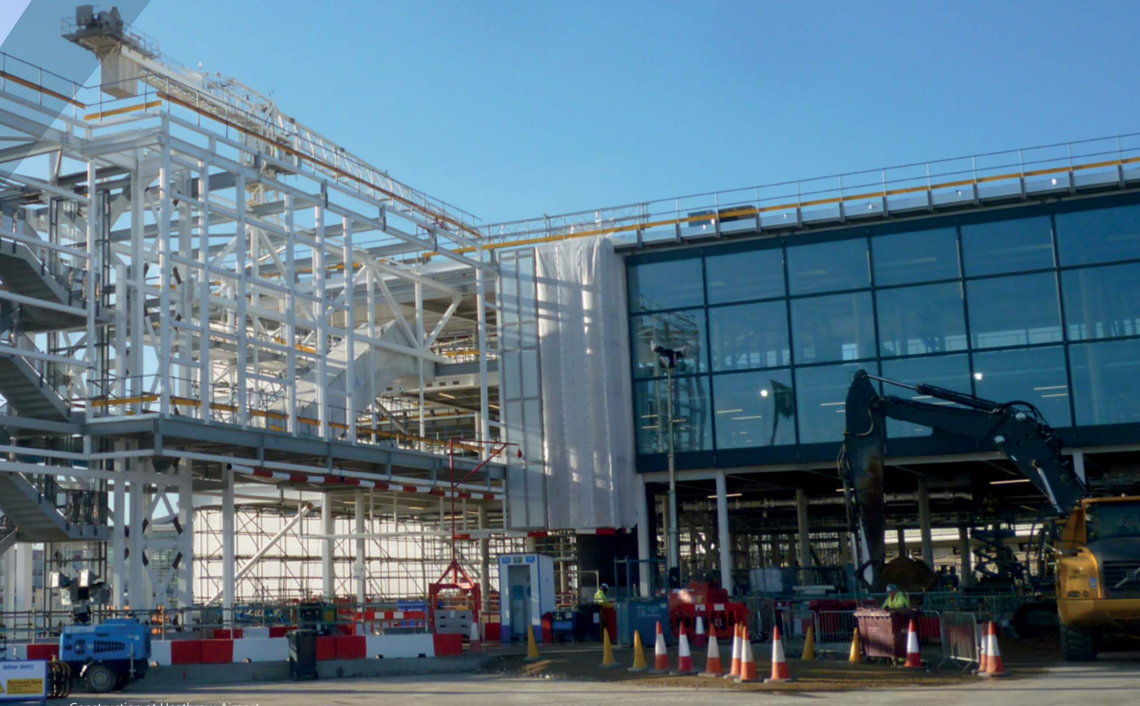
Construction at Heathrow Airport
