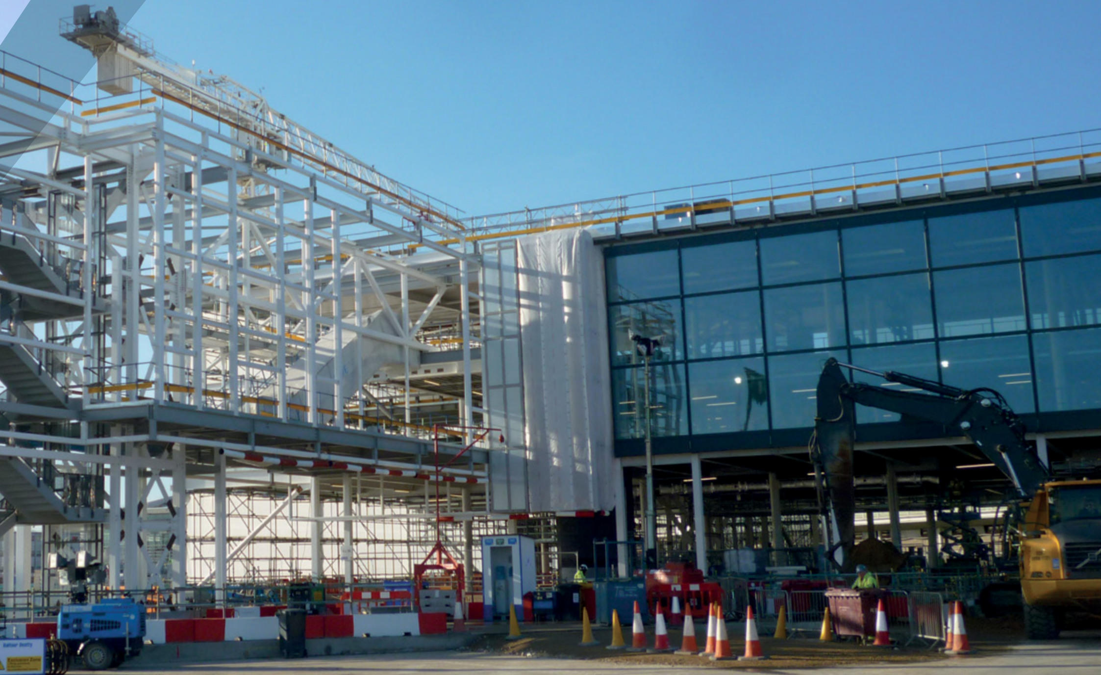
Construction at Heathrow Airport
