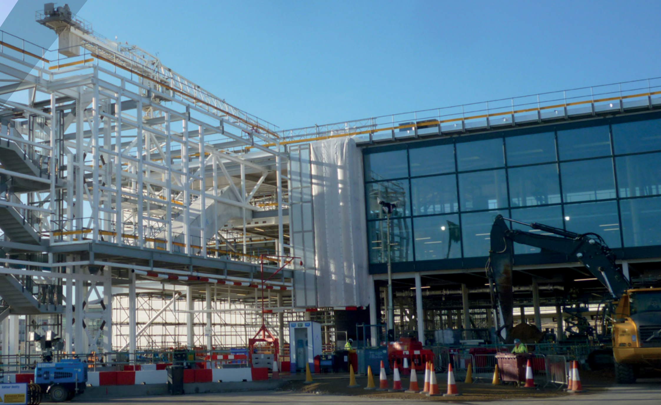
Construction at Heathrow Airport
