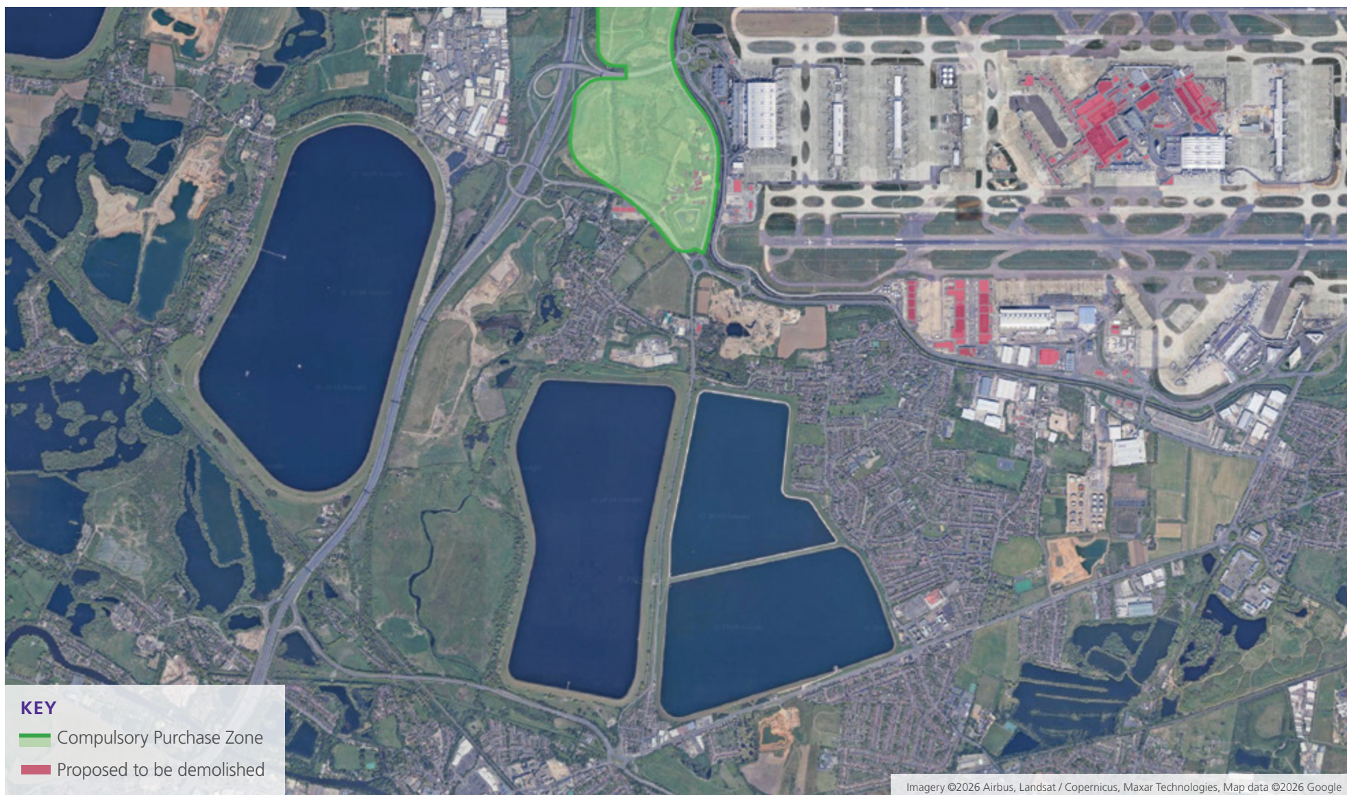
Aerial view of our proposed demolitions in Stanwell and Stanwell Moor
